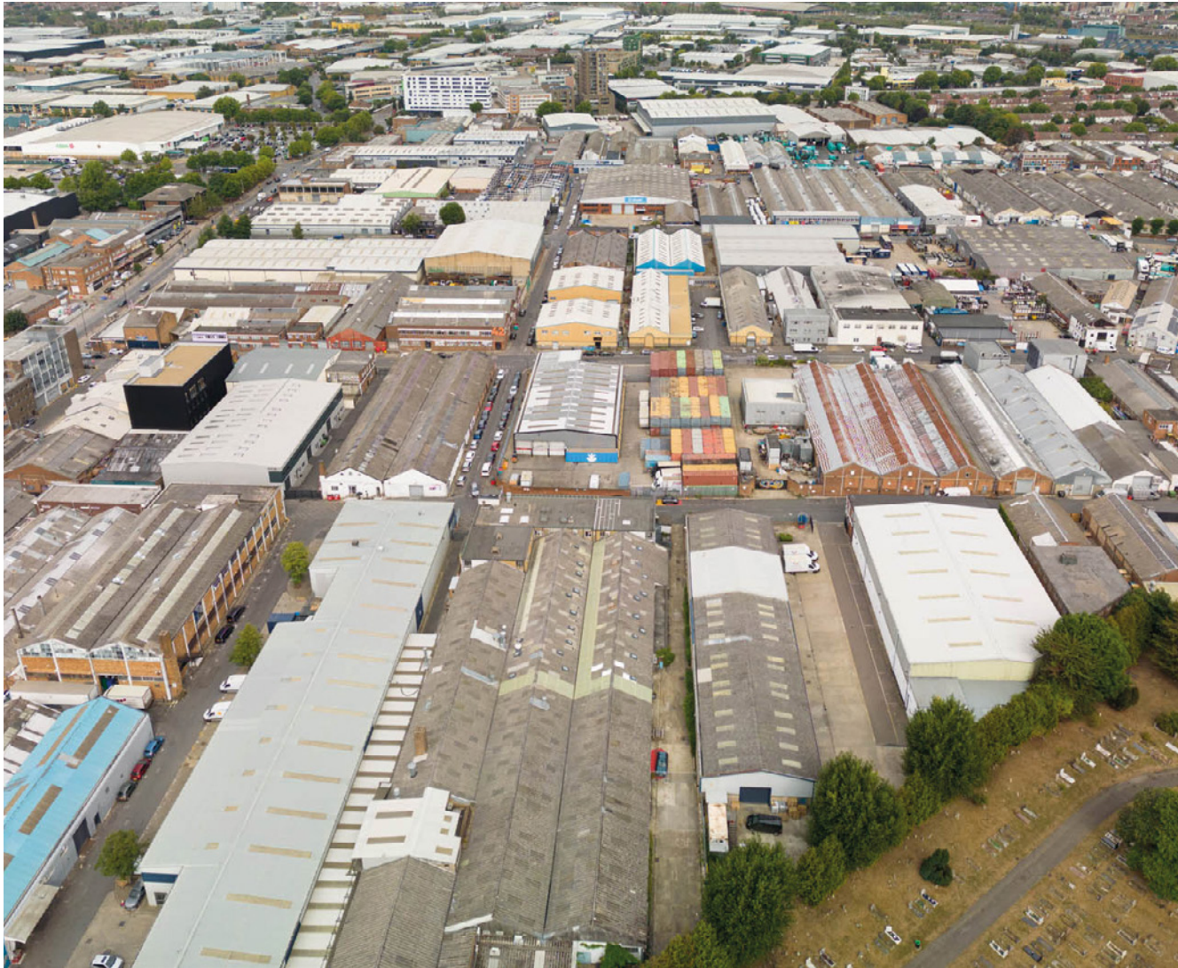
Image: Aerial view of North Acton Industrial Estate.
